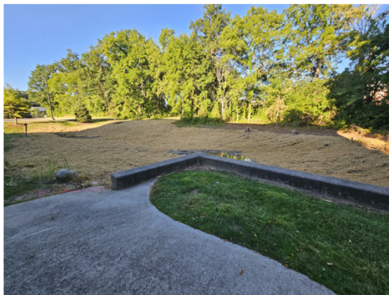
Restored retention pond
