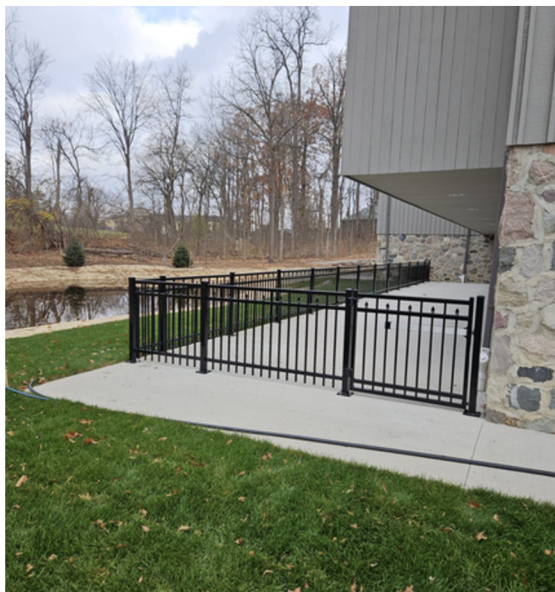
Patio, fence, and gate installation
