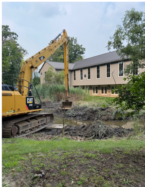
Retention pond dredging
